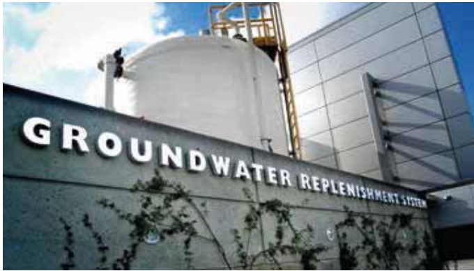
Groundwater replenishment system in Orange County, California, USA
